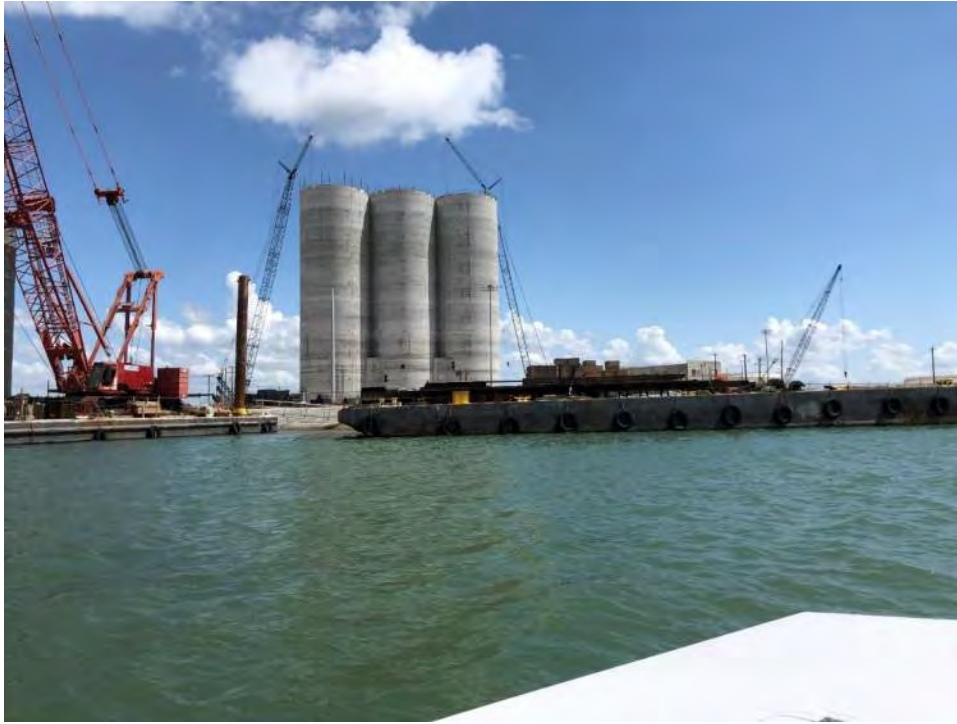
Photo 3- Photo showing northwest of proposed discharge location.
